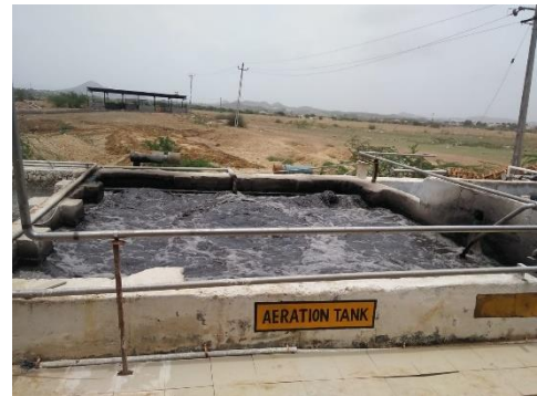
Figure 8: Aeration Tank
