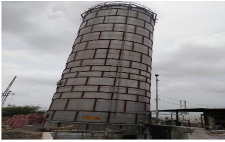
Figure 7: UASB Reactor
